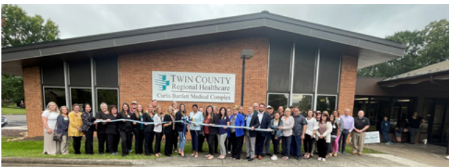
The newly renovated Curtis Bartlett Medical Complex houses our outpatient clinics for physical, occupational and speech therapy, orthopedics and cardiac rehabilitation.
